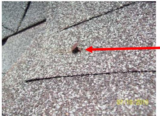
Flashing on the south and east side needs to be nailed down and sealed.
